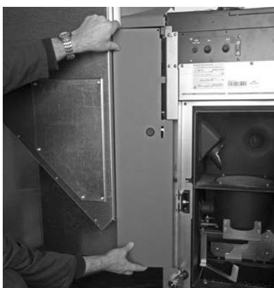
Fig.34 Insert front cladding
