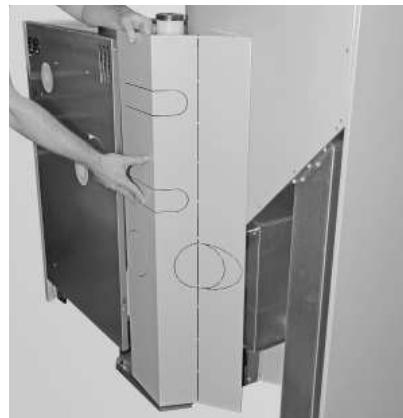
Fig. 28 Hook up cladding
