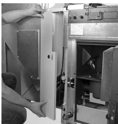
Fig. 33 Insert front cladding
