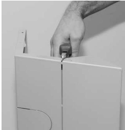
Fig. 25 Cut through lever at top and bottom
